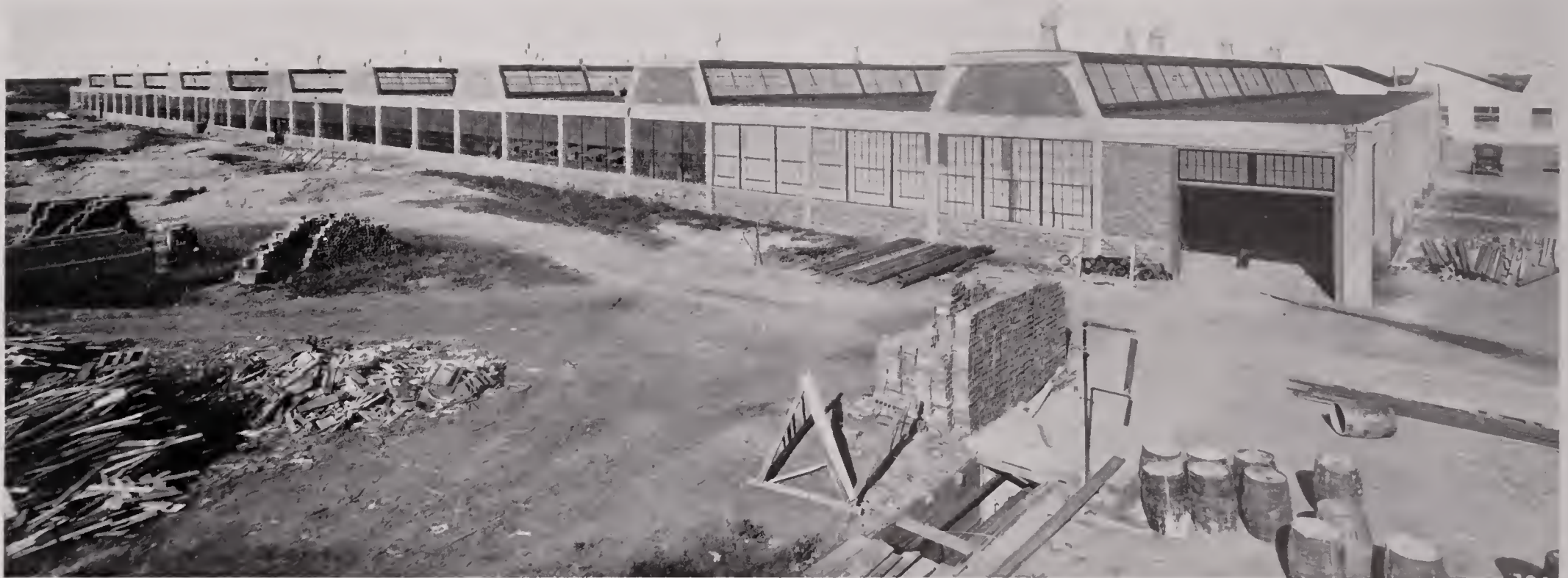
VIEW OF MAIN PRODUCTION UNIT FROM WEST SIDE
